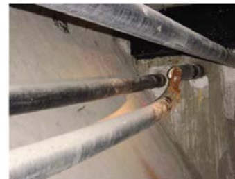
In May bridge inspectors discovered that one of the tendons beneath
