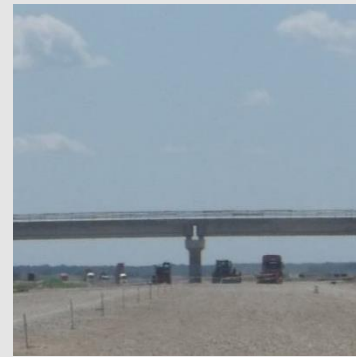
Bridges, decks and support structures
