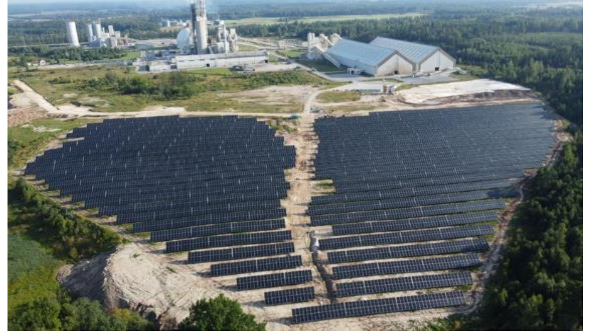
Internal park, 5 MW line (6.50 MW total)
