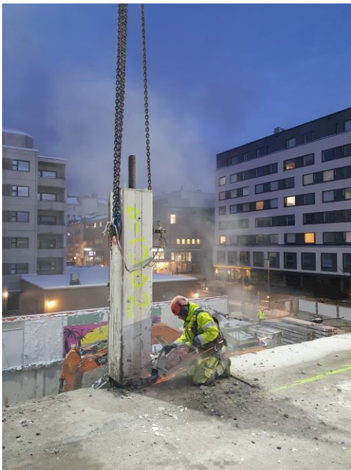
Figure 31. Lifting by drilling holes in the elements (wall and floor) and treading a chain or a slir through the holes (or in the case of columns, a lifting pin – not shown in the images). (Source Christoph Henschel, BTU [left] and Ramboll [right]).
