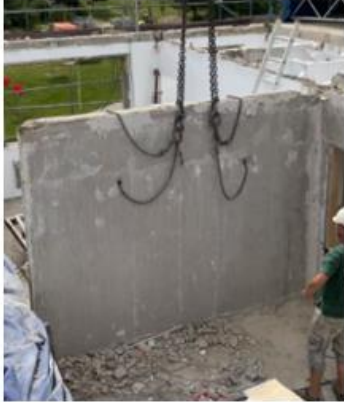
Figure 31. Lifting by drilling holes in the elements (wall and floor) and treading a chain or a slir through the holes (or in the case of columns, a lifting pin – not shown in the images). (Source Christoph Henschel, BTU [left] and Ramboll [right]).
