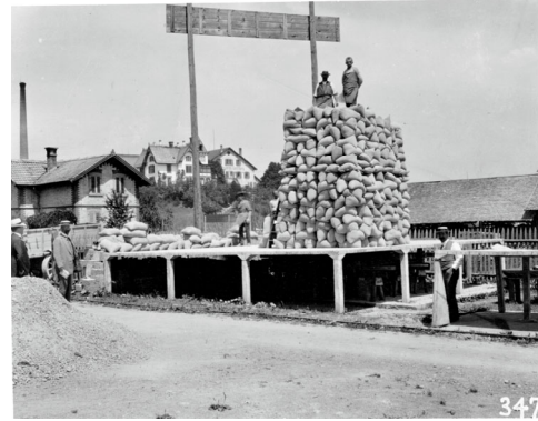
Photo: ETH-Bibliothek Zürich, Bildarchiv, Slab and beam tests, Joistless ceilings (mushroom ceilings). 1908
