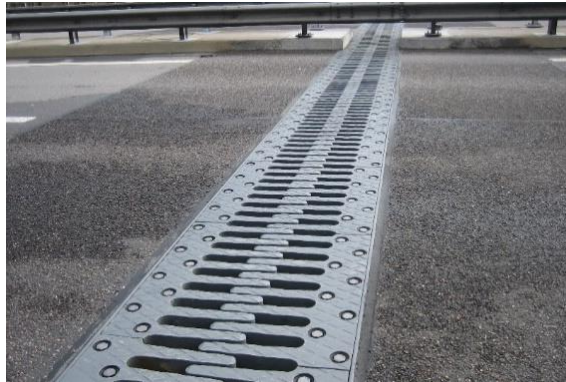
Cantilever finger joints
