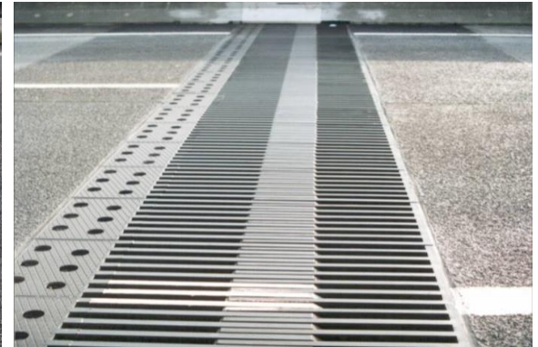
Sliding finger joints
