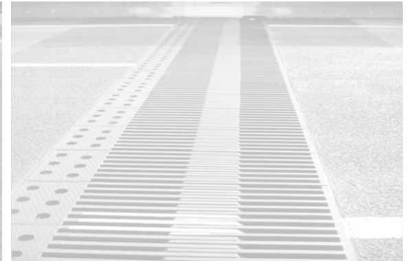
Sliding finger joints
