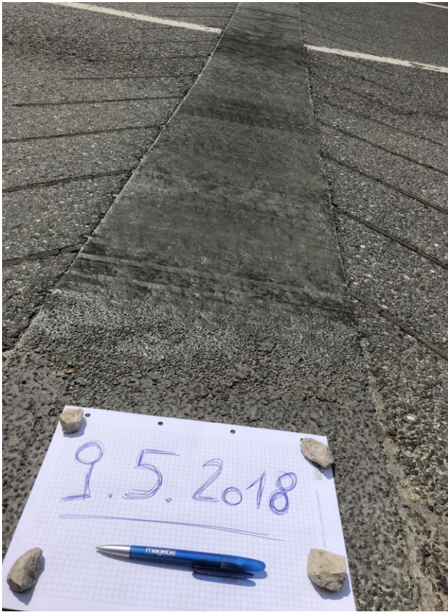
Austria – main road Obj. B25.06, PA 30, installation 2010
