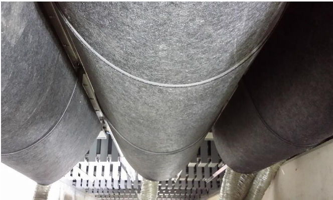
Lower side of noise barrier underneath the joint open
